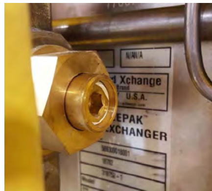
V3 INDICATOR OPEN POSITION
